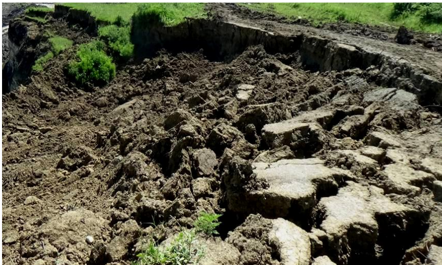
Figure 2. The upper left side of the landslide (detachment area)
