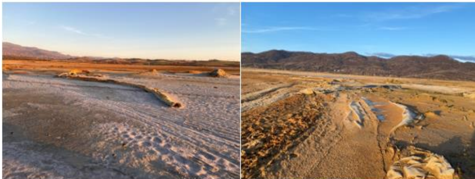
Photo 1. Degradation status of rehabilitation works
