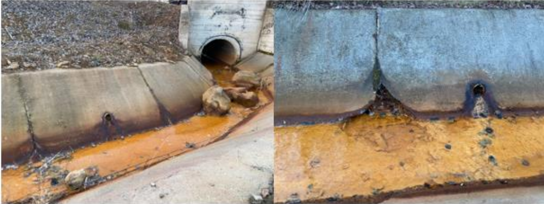
Photo 3. Acid drainage at the base of the pond where the perimeter gutter was arranged (concrete degradation and clogging of the drainage system)
